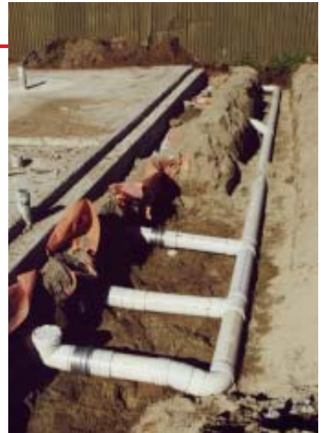
Main Sewer Drain under construction
